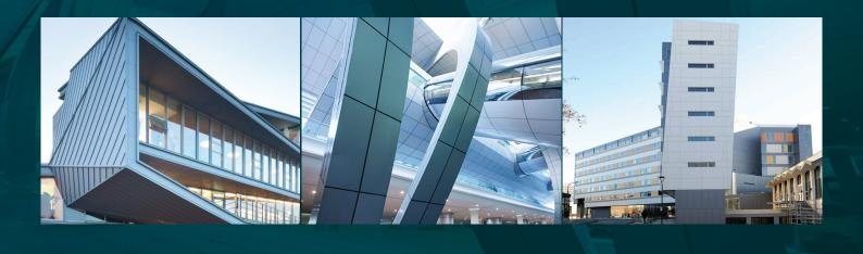
PROCORE A1° is a superior, DtS non-combustible, construction grade panel with a unique profiled aluminium core and a durable coating, making it an exceptional exterior cladding choice. PROCORE A1° is deemed to satisfy non-combustible when tested to AS 1530.1 and AS 1530.3 in accordance with the BCA/NCC requirements.
